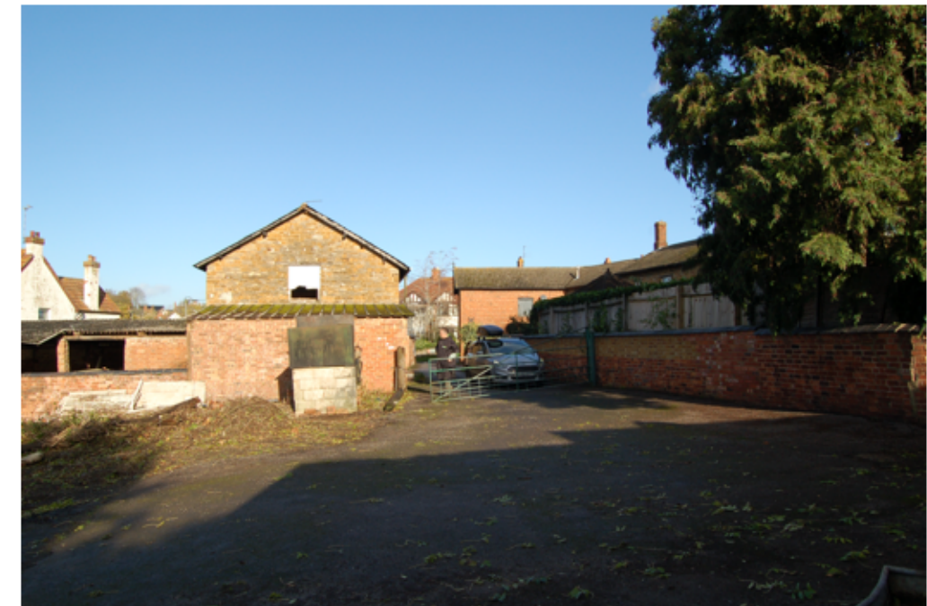
PS-001 F Gated site access point (right), looking north towards Broad Street.
