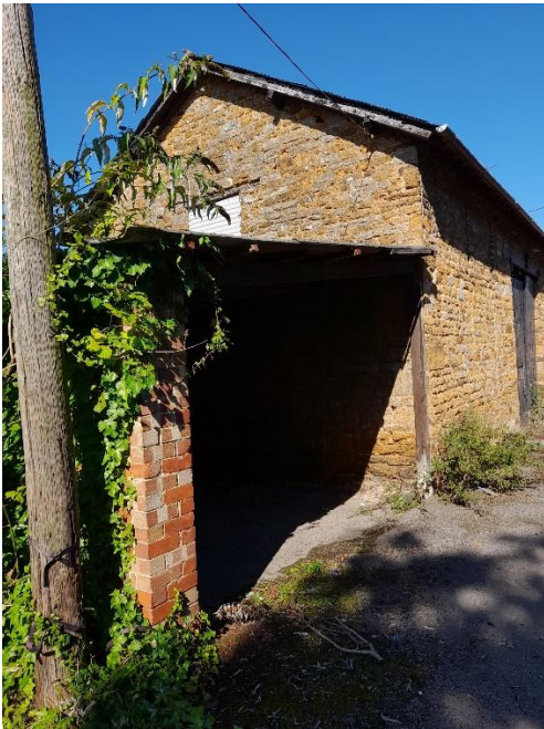
Fig 2. Barn exterior, south gable with modern lean-to (to be removed).
