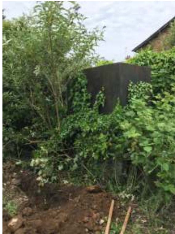
Above-ground oil tank to south of Plot 4 – 23 rd May 2023
