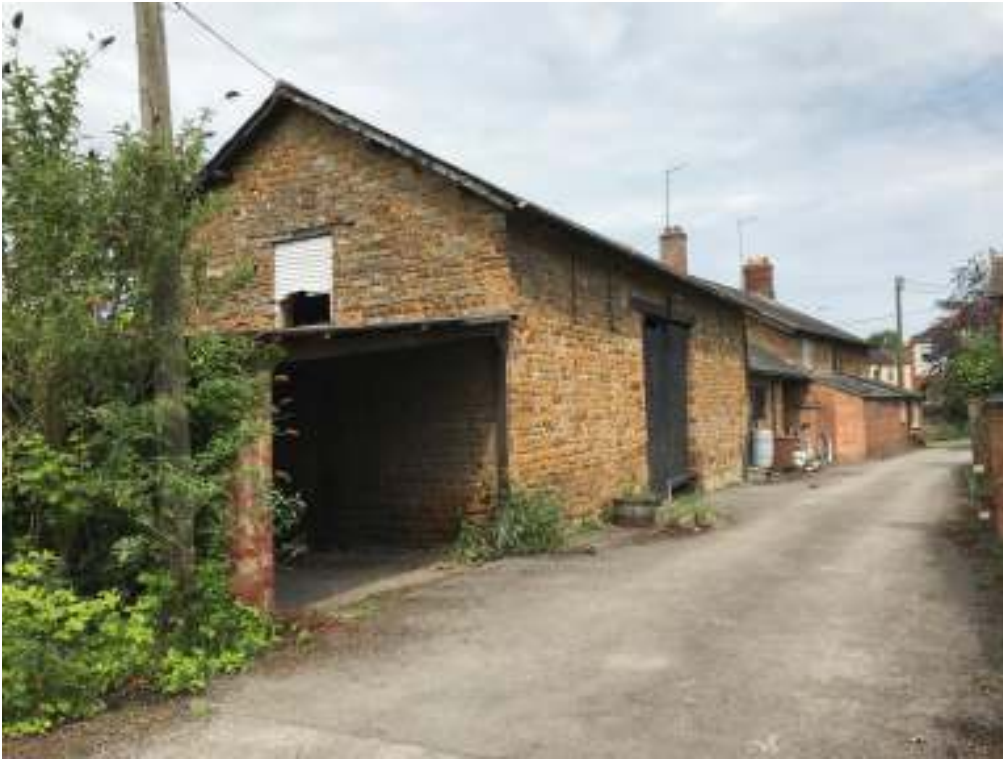
Barn (Plot 4) to be converted - 23 rd May 2023
