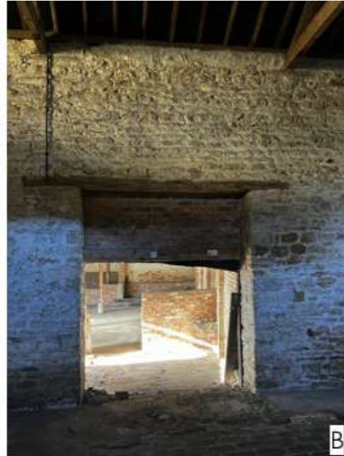
Link to covered area with feeding troughs (west)
