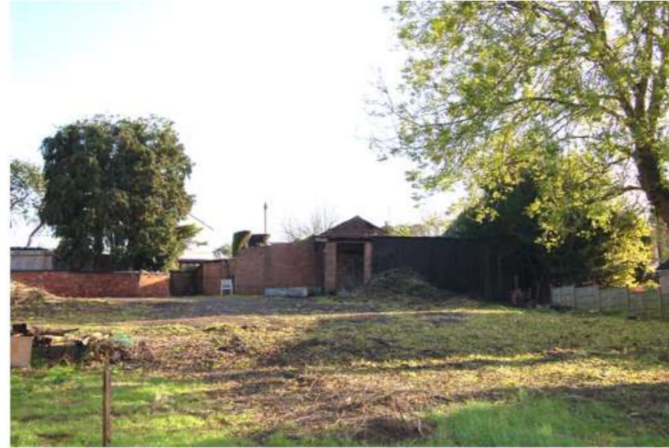
PS-002 B View from within the site looking east with the outbuildings surrounding the Smithy in the distance.
