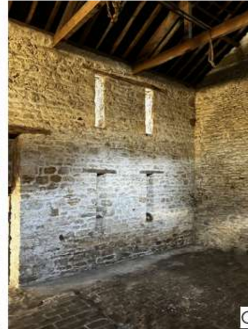
Openings on the west facing elevation.
