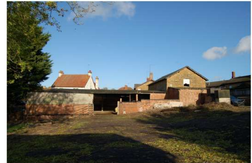
PS-002 F Northerly view from within the site, looking towards the covered shelter area that is situated to the west of the Stone Barn.
