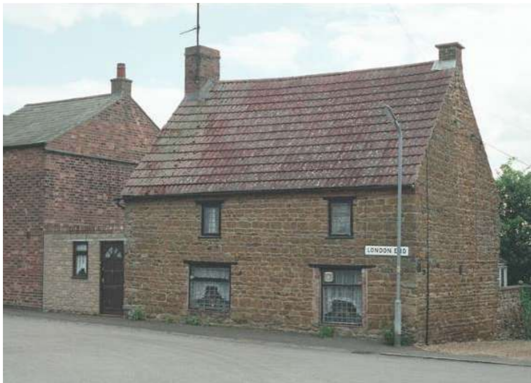
Listed Building. The Cottage, 2 London End, Earls Barton.
