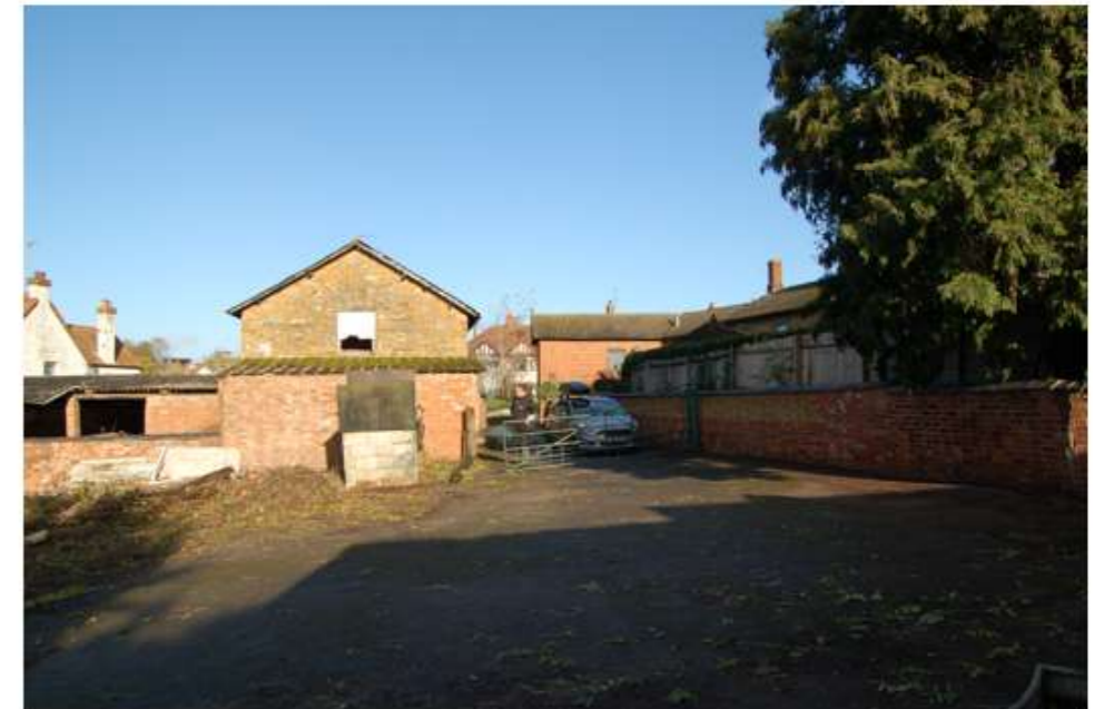
PS-001 F Gated site access point (right), looking north towards Broad Street.
