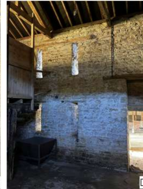
Openings on the west facing elevation.
