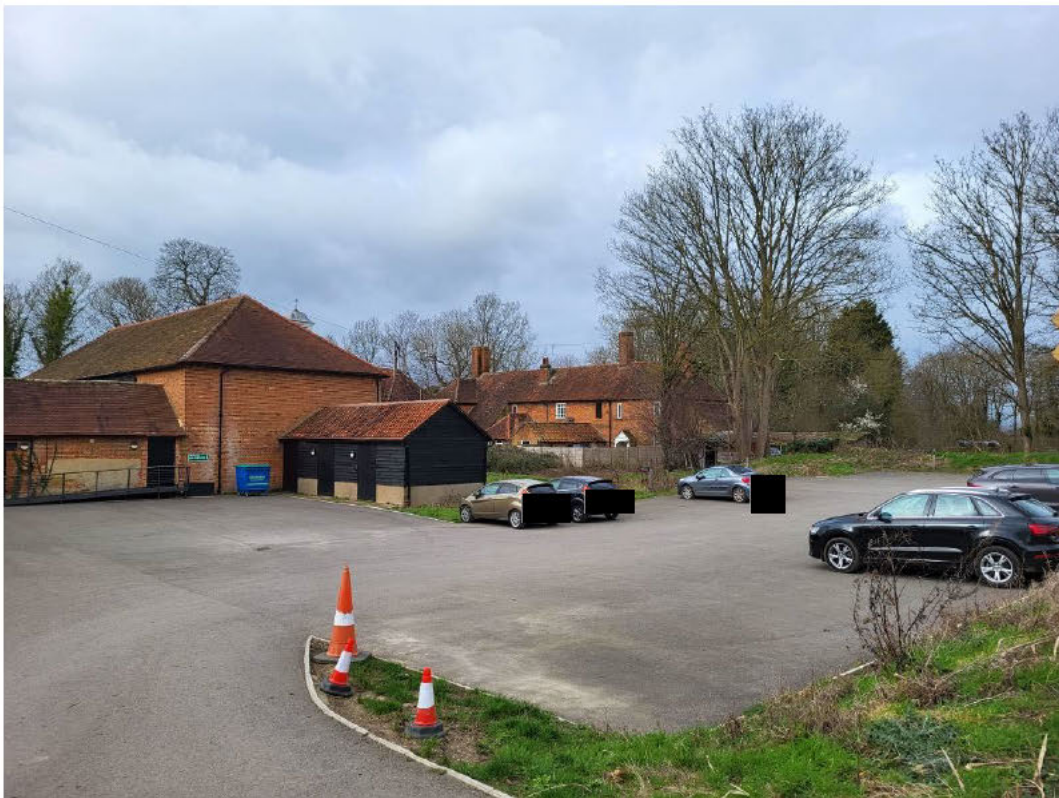
Plate 20: Looking north-west across former farmyard towards listed Place Farm buildings
