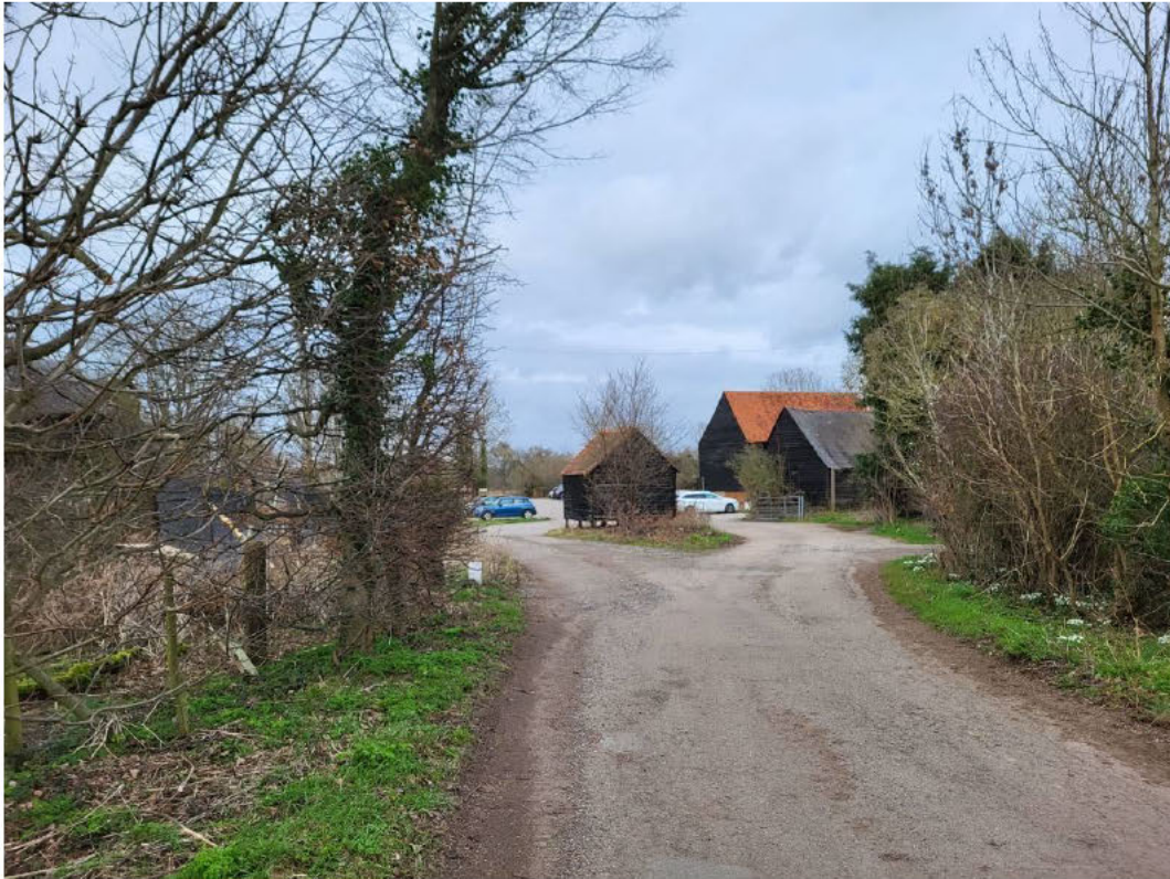
Plate 17: Looking north from top of Place Farm driveway into the eastern former farmyard area (unlisted granary in centre and listed barn to right)
