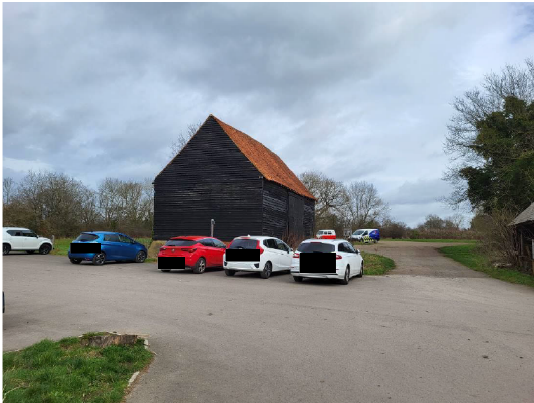
Plate 25: Looking east across former farmyard to listed three-bay former threshing barn
