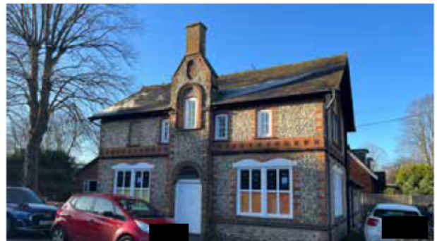
Former school house, Ockham Road South
