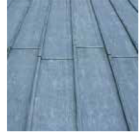
Lead roll flat roof
