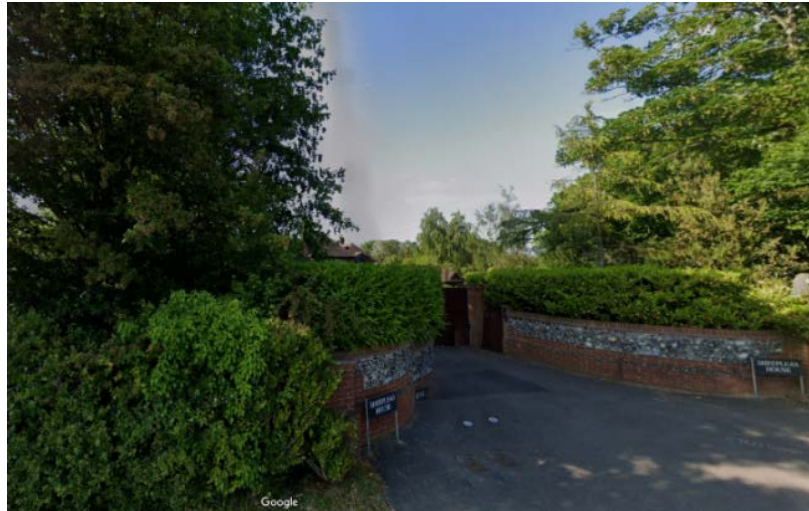
Photos detailing the entrance gates and boundary walls
