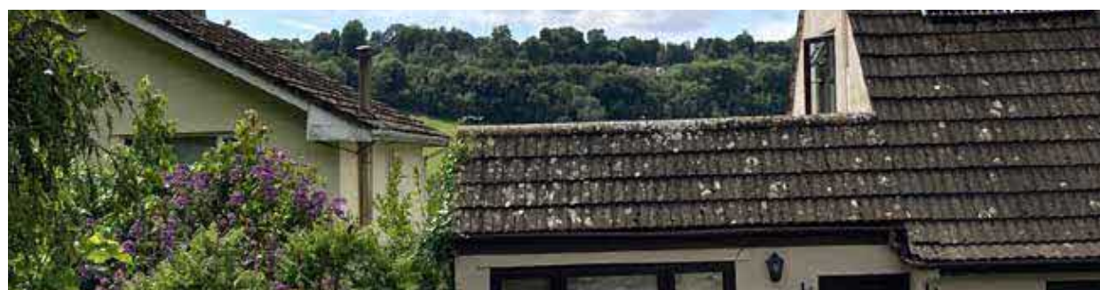
Existing single-storey outshot with 'faux' roof connected to the main bungalow
