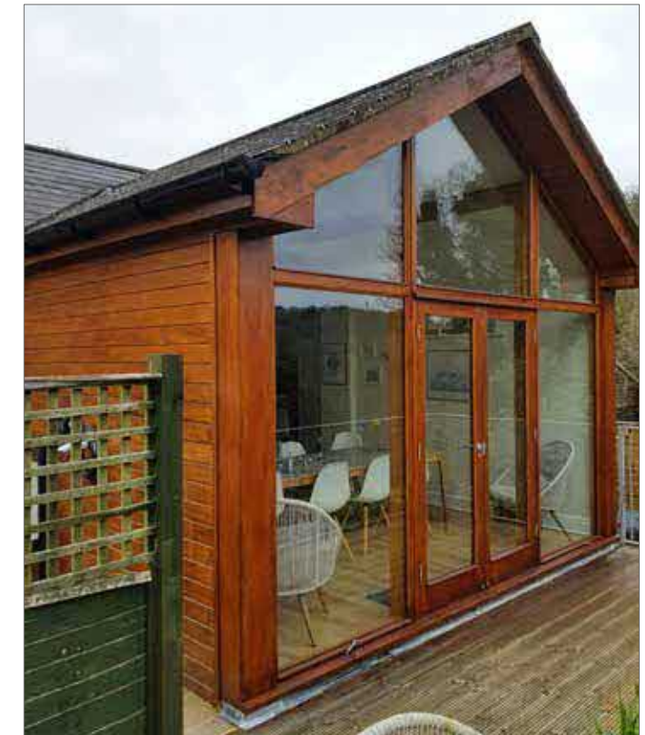
'The Old Stables' - contrasting extension towards views
