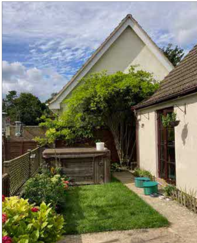
Neighbour's gable wall ('Fairbourne') to north
