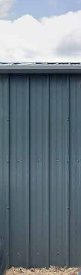
Grey profiled metal cladding to match existing show room
