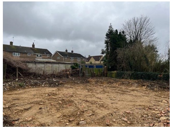
View towards Rear ( north ) Boundary
