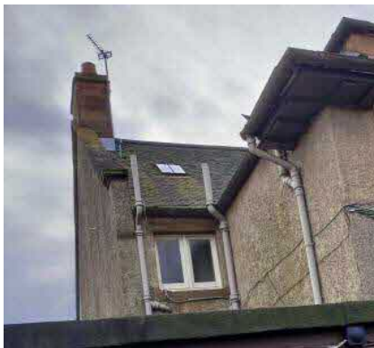
Existing WC Window
