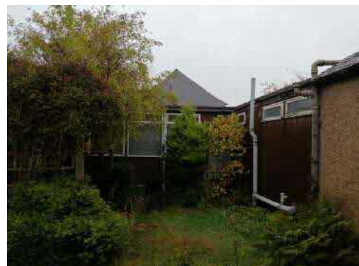
Existing NE Extension - Windows
