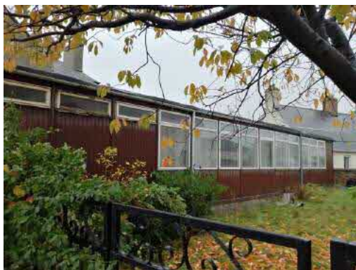
Existing NE Extension - Windows
