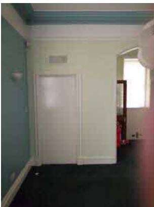
29. Previous blocked up opening to GFL
