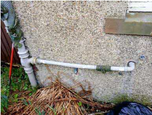
19. UPVC waste branch to annex
