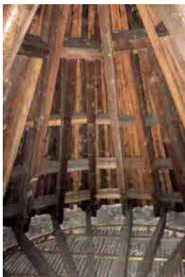
7. Roof void - turret
