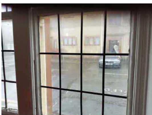
15. Plain glass overlay with insulating tape
