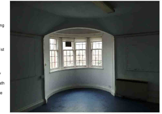
Extract Fan Cored Through Window
