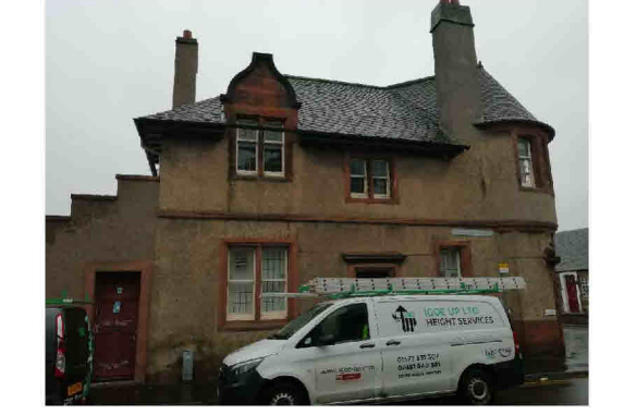
Side (SW - Douglas Cres Elev - RHS)
