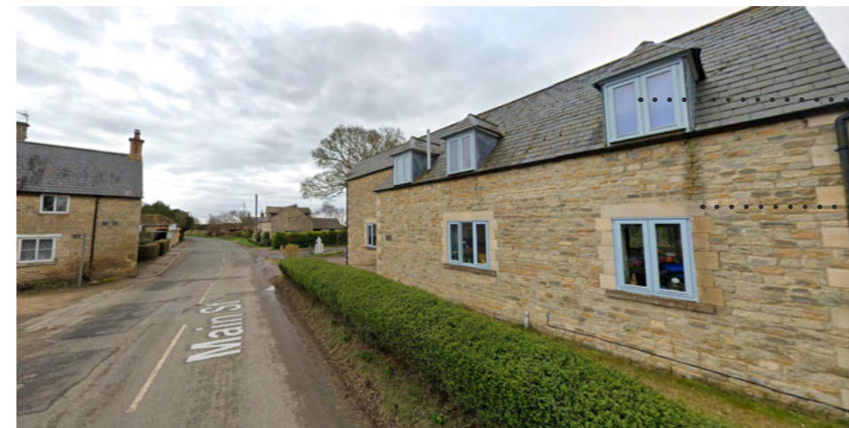
•••• Hipped dormer windows with painted timber casement windows
