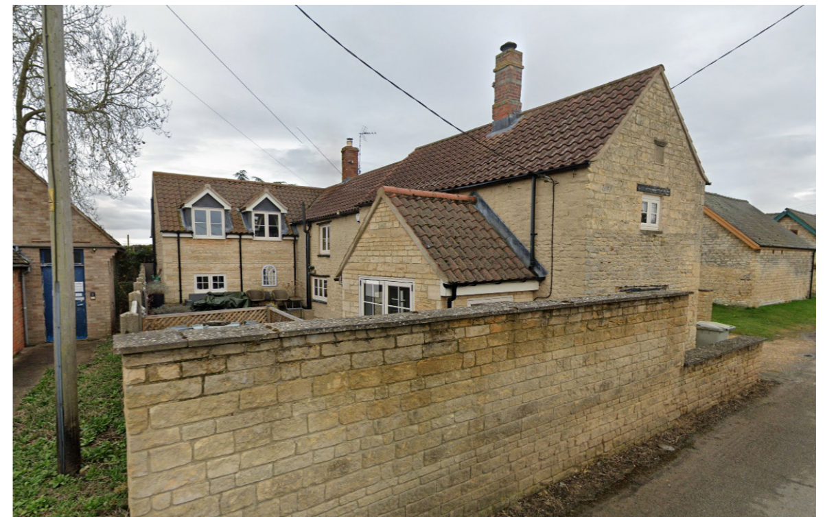
An example of a property with single, 2 and 1.5 storey elements and an additional porch at the front. Creating varied roof heights
