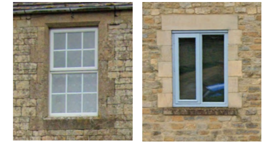
Sash and casement windows with stone surround
