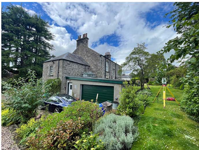
PHOTO 9. VIEW OF RAISED GROUND TO REAR, SHOWING EXISTING GARAGE SET WITHIN HIGHER GROUND.
