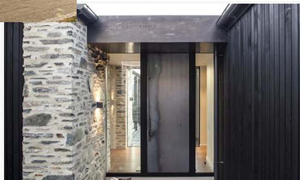
CHARRED/ DARK TIMBER CLADDING ADJACENT TO NATURAL STONE
