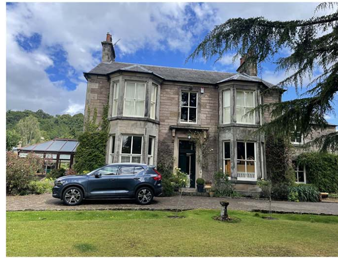
PHOTO 3. FRONT ELEVATION, SHOWING CONSERVATORY TO WEST.
