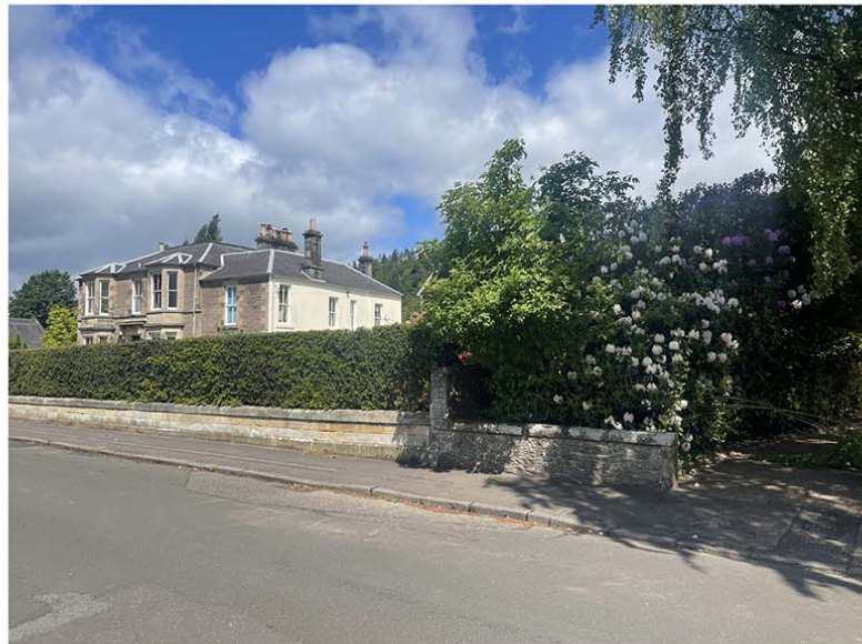
PHOTO 5. EXISTING PROPERTY TO WEST
