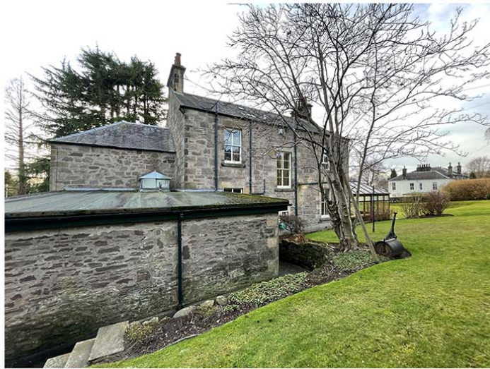
PHOTO 5. VIEW OF NORTH ELEVATION, OBSCURED BY EXISTING GARAGE
