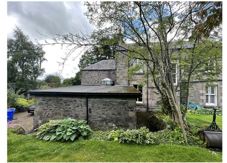
PHOTO 4. REAR ELEVATION LOOKING AT NORTH ELEVATION OF GARAGE.
