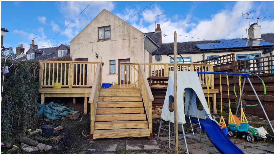
Figure1: Decking and Steps as Existing
