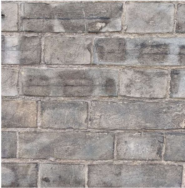
Existing Suffolk White bricks
