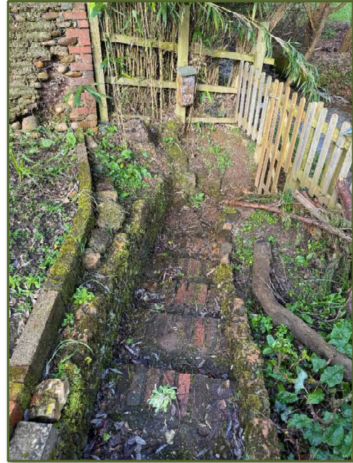
Figure 9: Hard landscaping to be made good.
