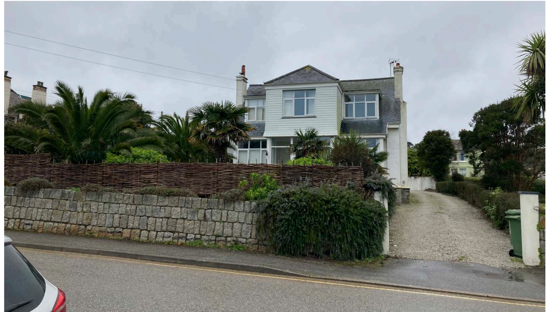
Existing street view
