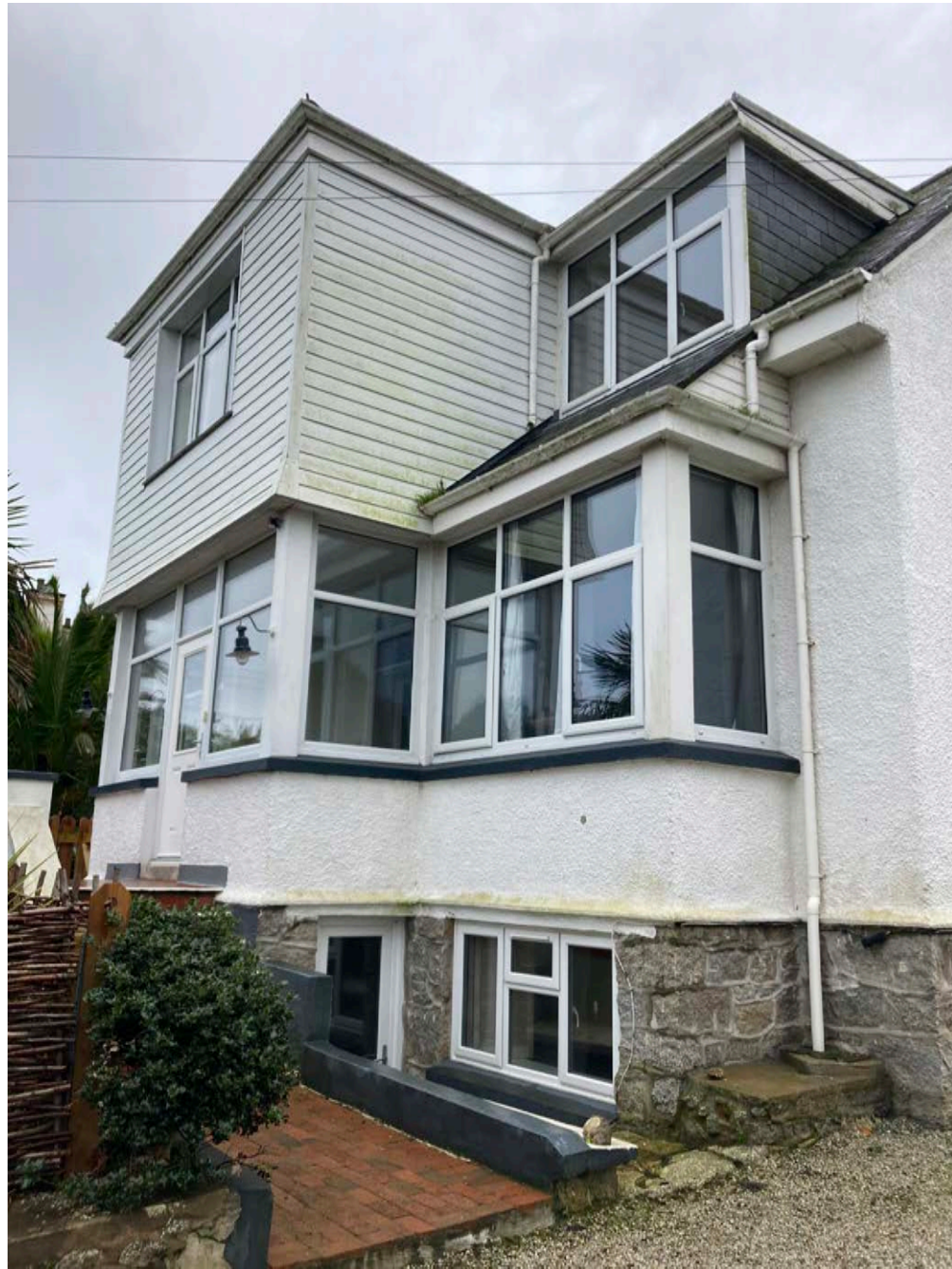
View at property north-east corner
