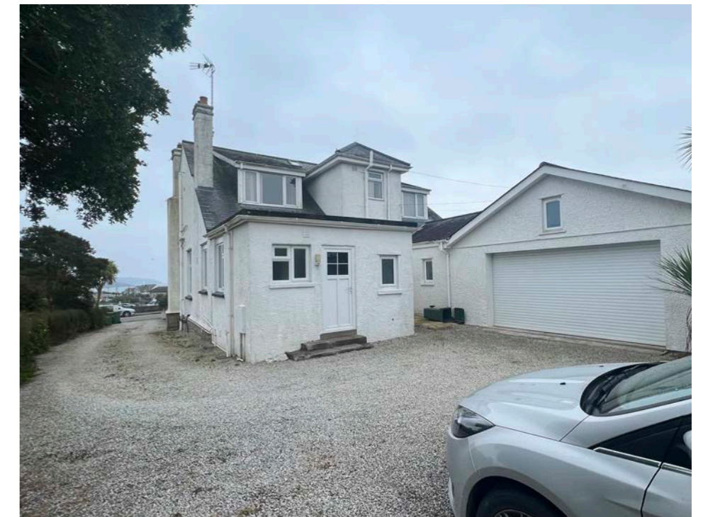
Existing view from rear parking area
