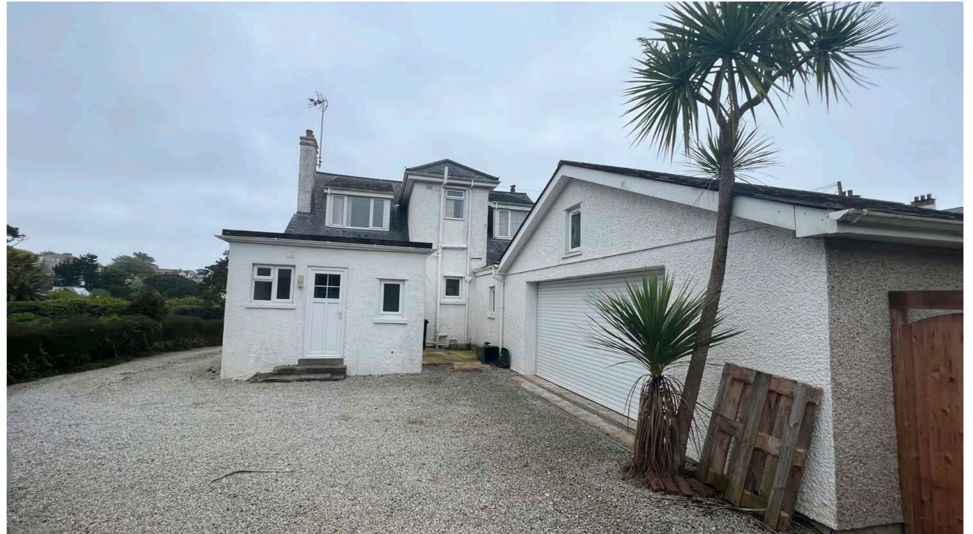
Rear view showing existing parking area and rear entrance
