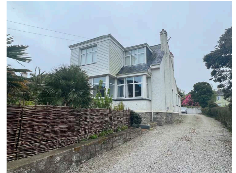
Existing view from driveway entrance
