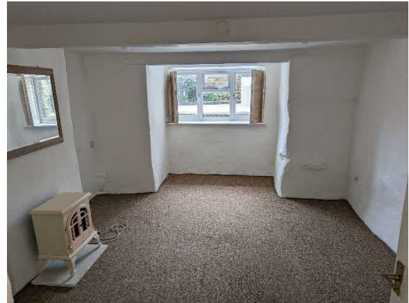
Photo 8. Showing the basement
