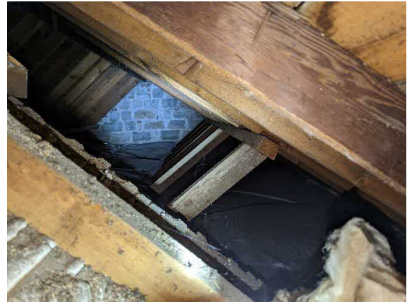
Photo 6. Showing the southern part of the roof void over the house
