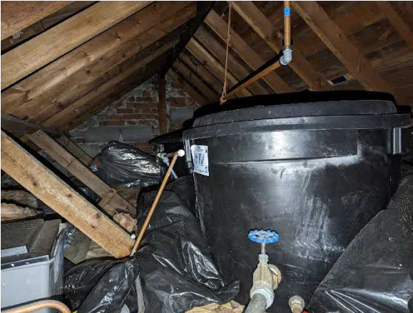
Photo 5. Showing the northern part of the roof void over the house
