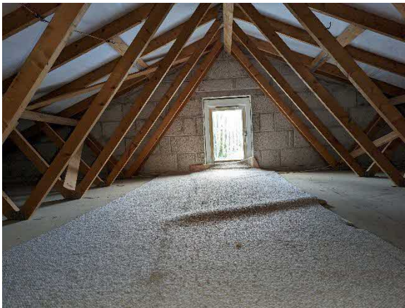
Photo 7. Showing the roof void over the garage
