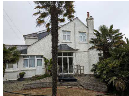
Photo 2. Showing the house from the south
