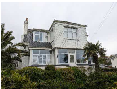
Photo 1. Showing the house from the east
