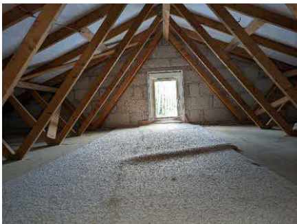
Photo 7. Showing the roof void over the garage
