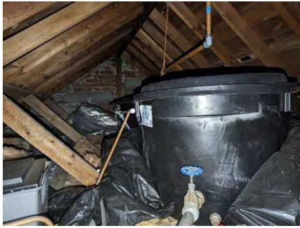
Photo 5. Showing the northern part of the roof void over the house
