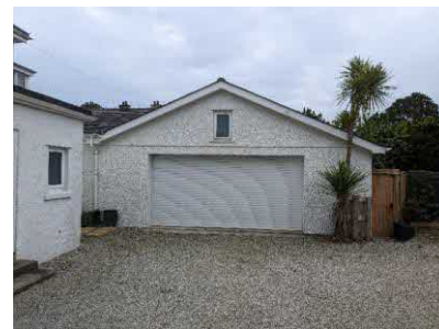
Photo 4. Showing the garage from the north
