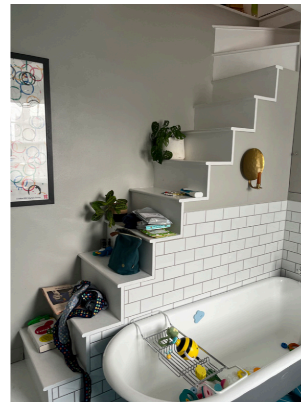
Existing family bathroom with stairs to loft
