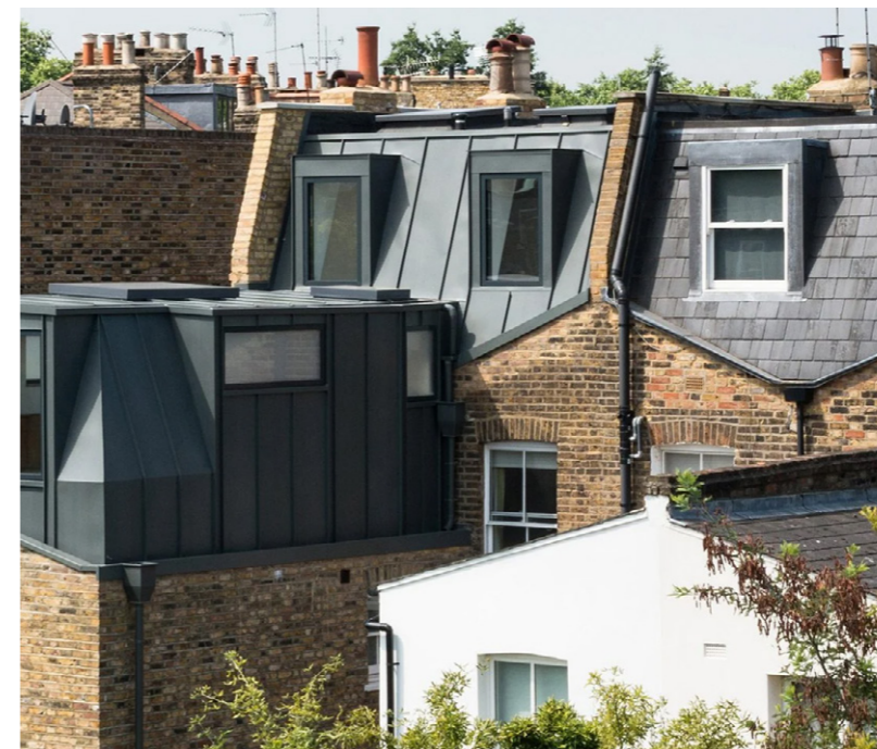
Zinc loft extension with slim frame aluminium windows
