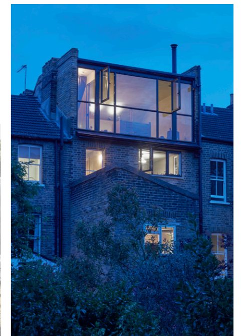
Parapet walls in London stock brick and slim frame glazing
