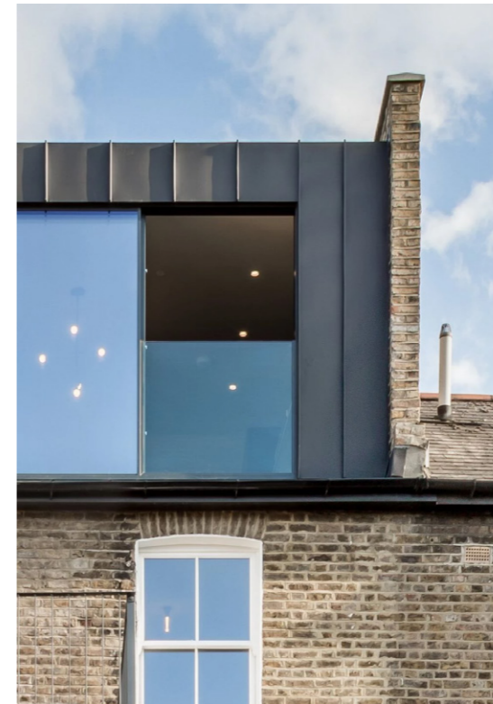
Sliding door and glass balustrade within zinc clad loft
