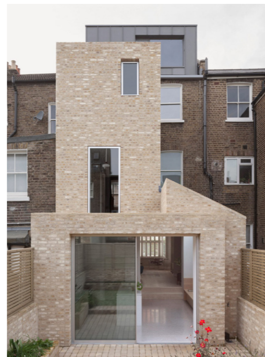
Simple zinc clad roof extension
