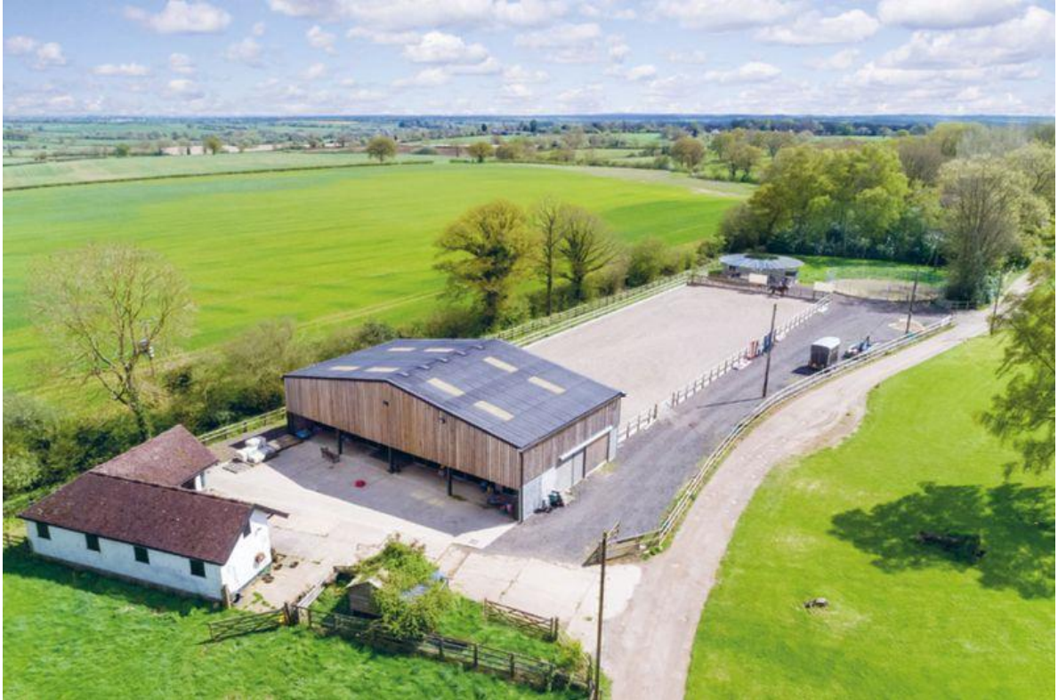
Figure 2: Aerial Photograph courtesy of Agents
