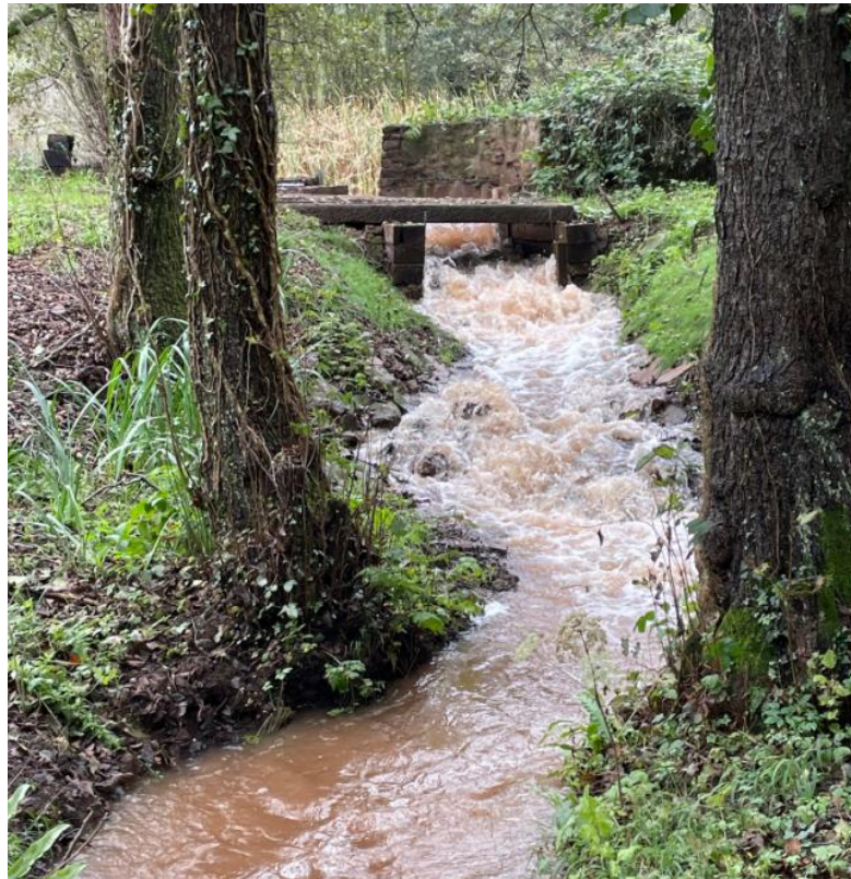
Figure: 13 Step Pool Cascade From Upper Pond Outlet
