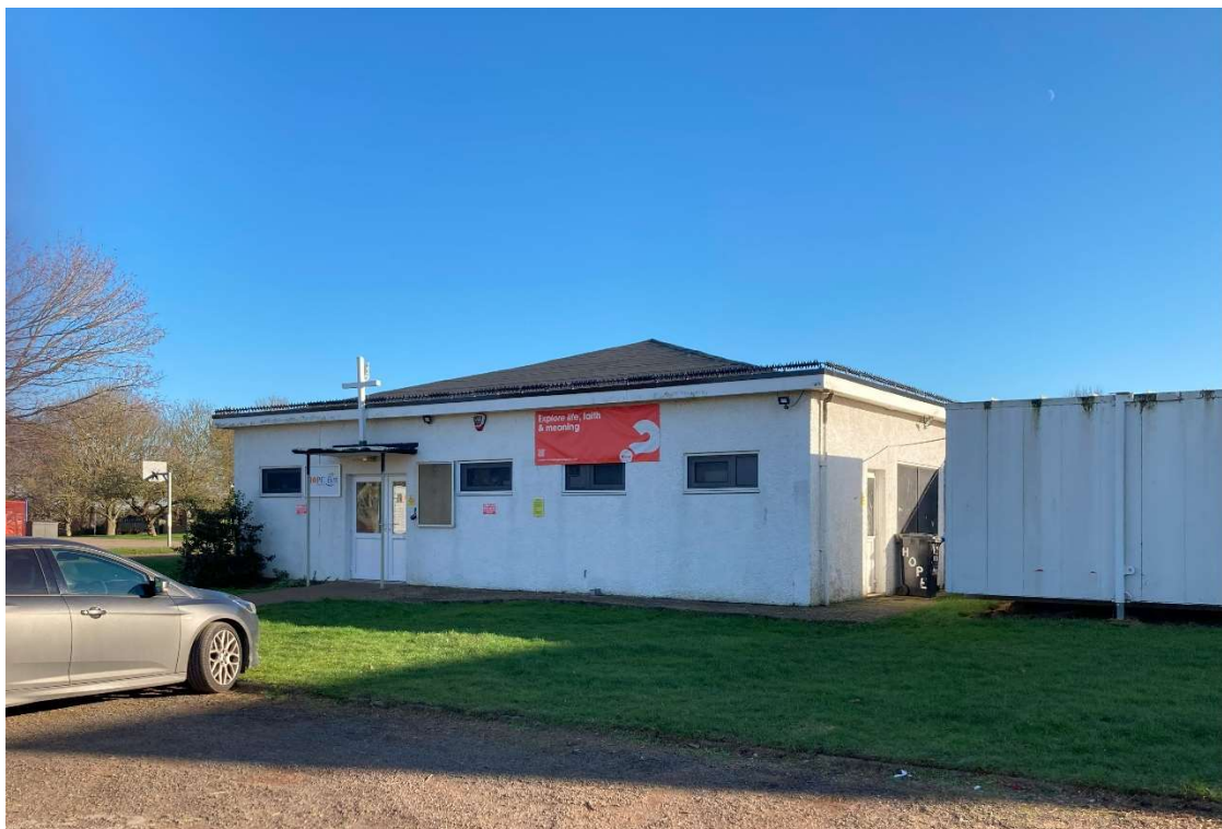
The Hope Church, Guillemot Lane, Wellingborough NN8 4UH
