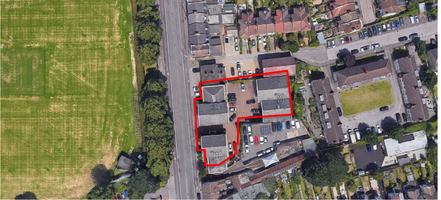
Figure 4: Aerial view of the site as existing
