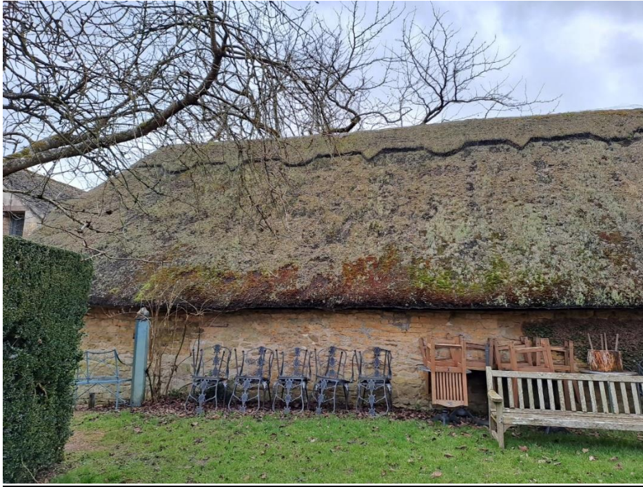
4. North Elevation, showing close proximity of Prunus tree
