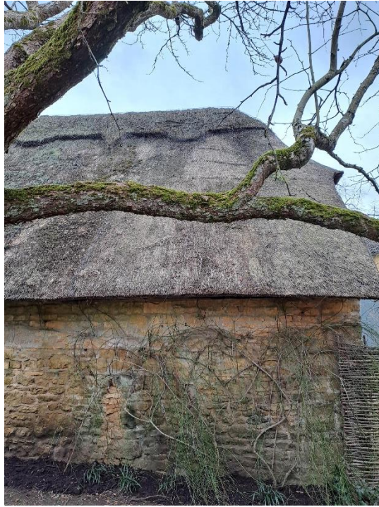
6. Eastern End of South Elevation
