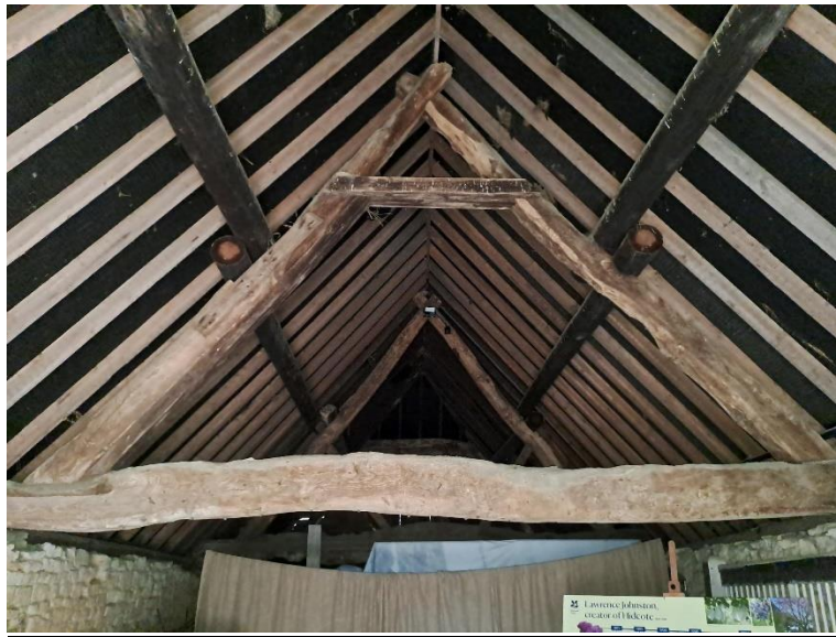
7. Internal view of roof timbers
