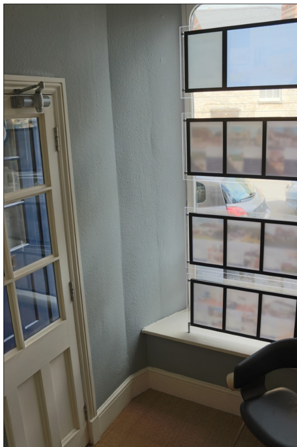
Plate 3: Internal view of the window and modern internal partition to left
