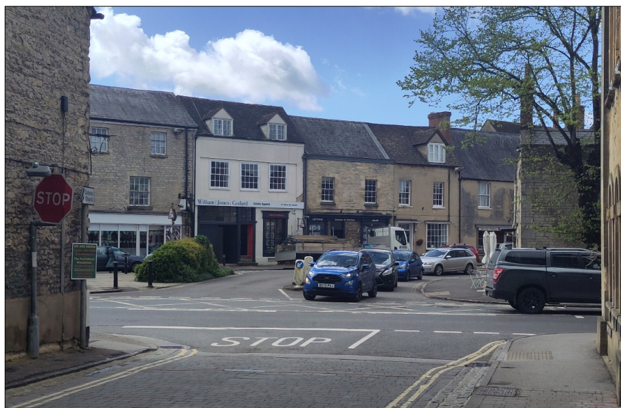
Plate 4: 34 High Street flanked by 32 High Street (to the right) and 36 (to the left)
