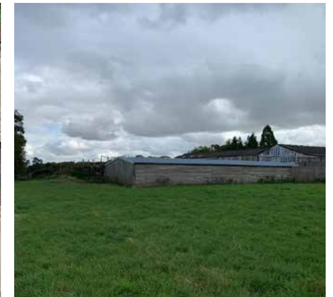
View of the proposed GSHP collector array location
