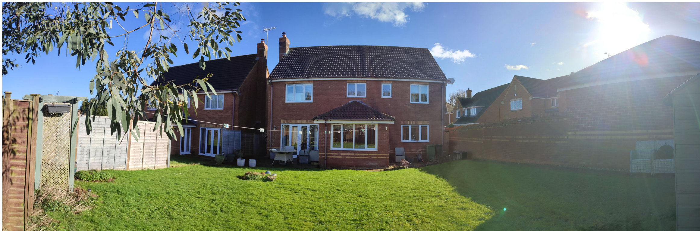
Existing Photo 2 - Rear elevation viewed from garden lawn
