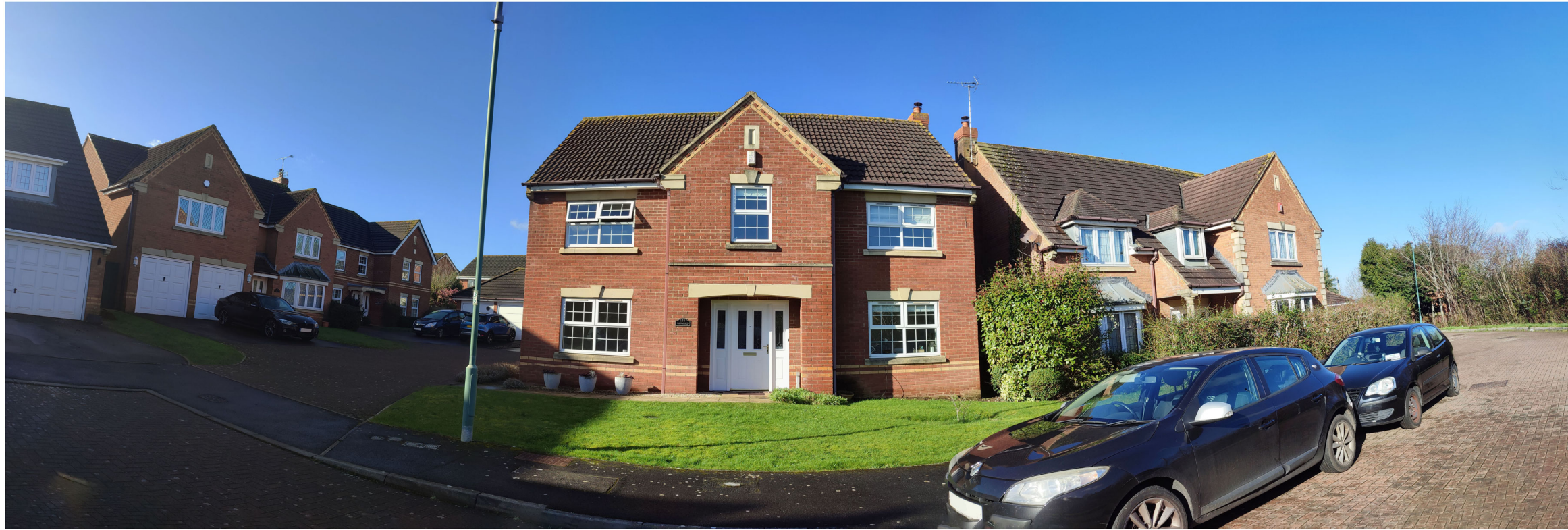
Existing Photo 1 - Front elevation
