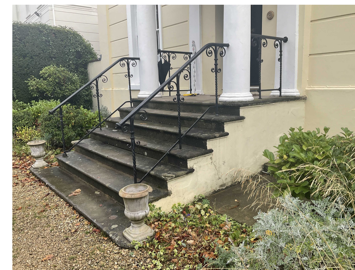
Existing steps and balustrade.
