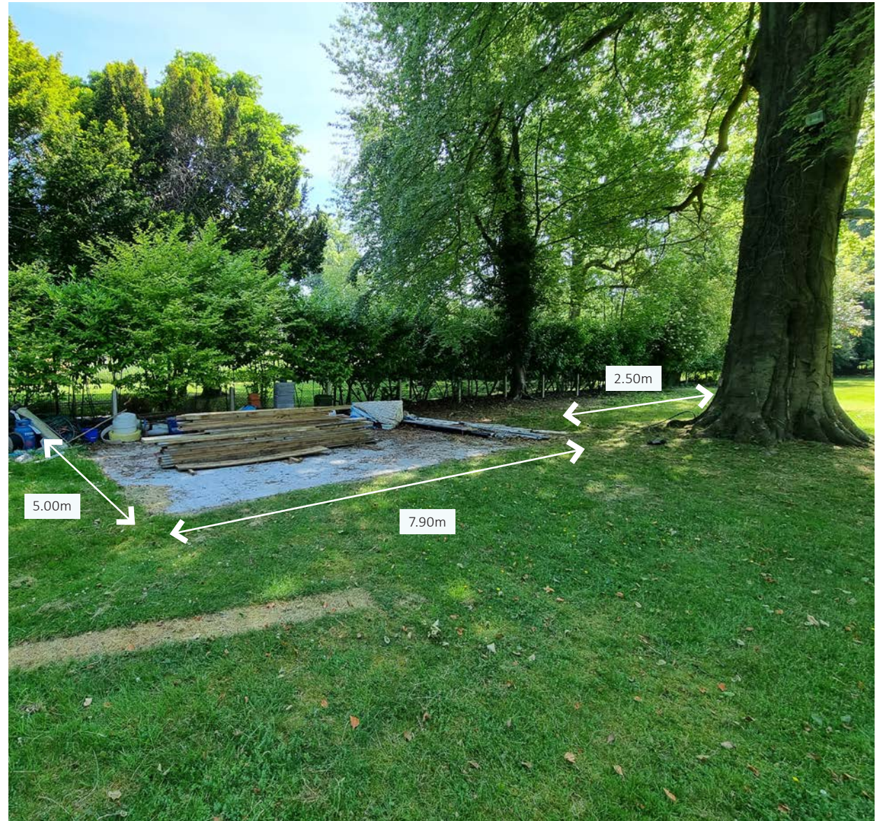
View of the existing concrete pad along the northern boundary
