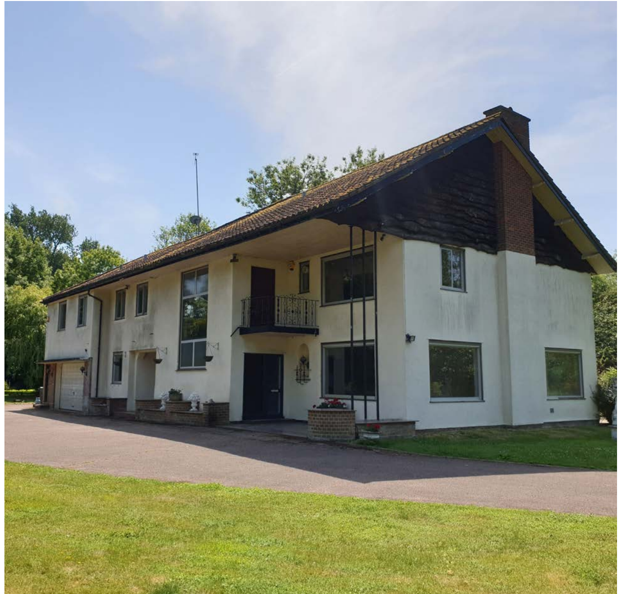
Existing building front elevation viewed from the River Chess prior the start of building works
