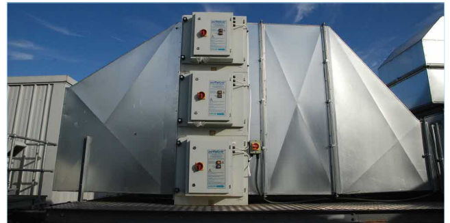
3 ESP Units Stacked in modular formation
