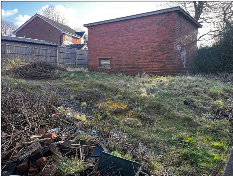
General view to south east of existing electrical sub-station
