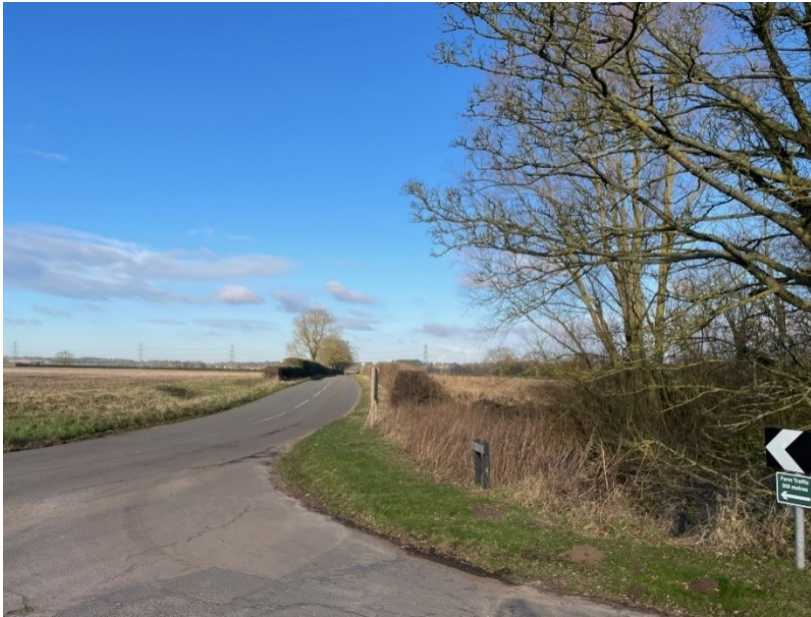
Photo 2.1: Southern Access Road (looking North)
