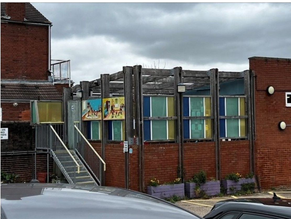
ELEVATED PLAY AREA AT ADJOINING SITE
