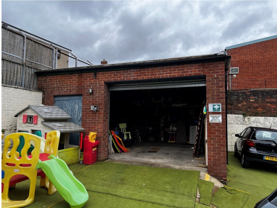
EXISTING EQUIPMENT STORE
