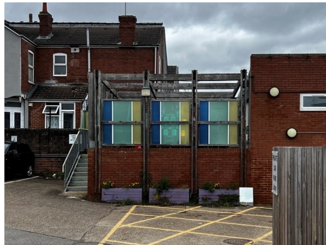
ELEVATED PLAY AREA AT ADJOINING SITE
