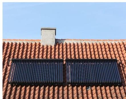
The space for solar thermal panels would be limited to the available roof space and it is likely that it will not be sufficient to meet the hot water demands. Additionally, the roof space has been utilised for PV to generate electricity and the carbon savings associated with solar thermal panels would be significantly less than PV.
