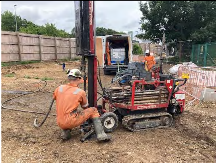
Injection works within plume area
