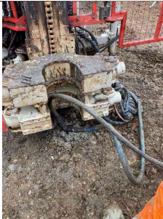
Grout injection during decommissioning of BH509
