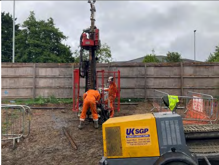
Over-drilling of BH402 for decommissioning
