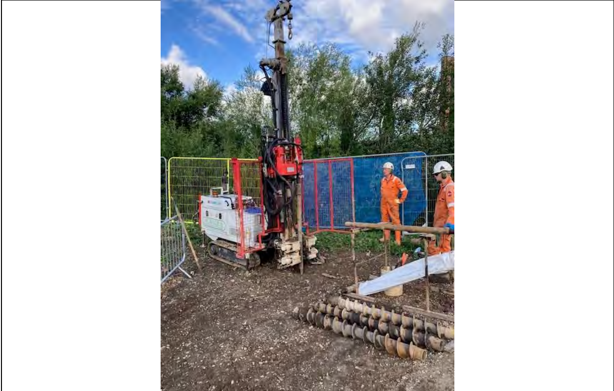
Percussive sampling of BH603
