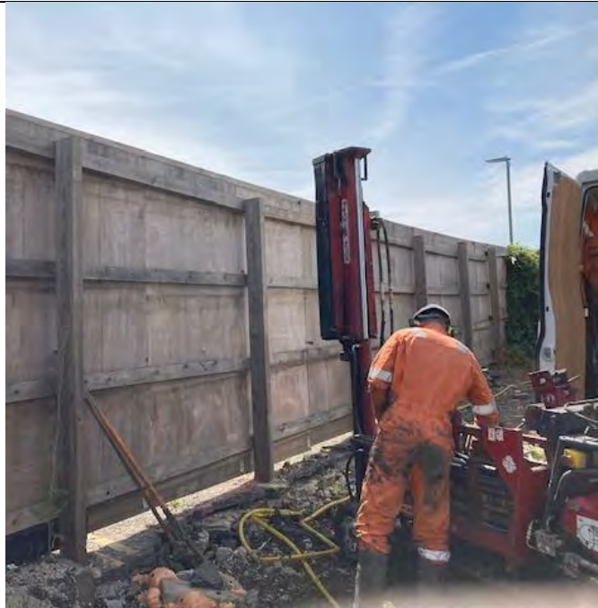
Injection works at barrier area adjacent to NE site boundary
