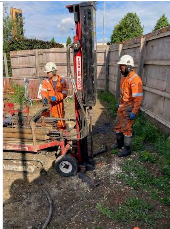
Injection works barrier area
