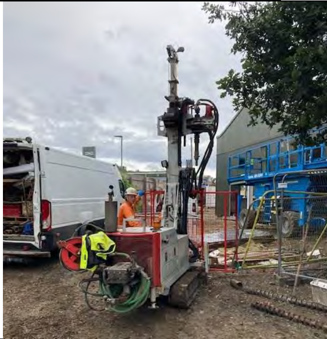
Decommissioning of BH403
