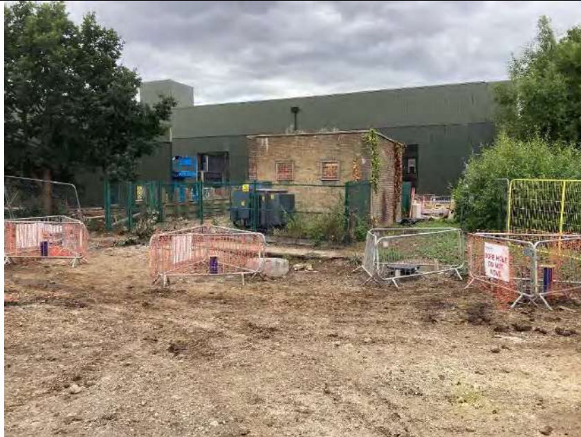
Final site area condition following injection, decommissioning and borehole installation works
