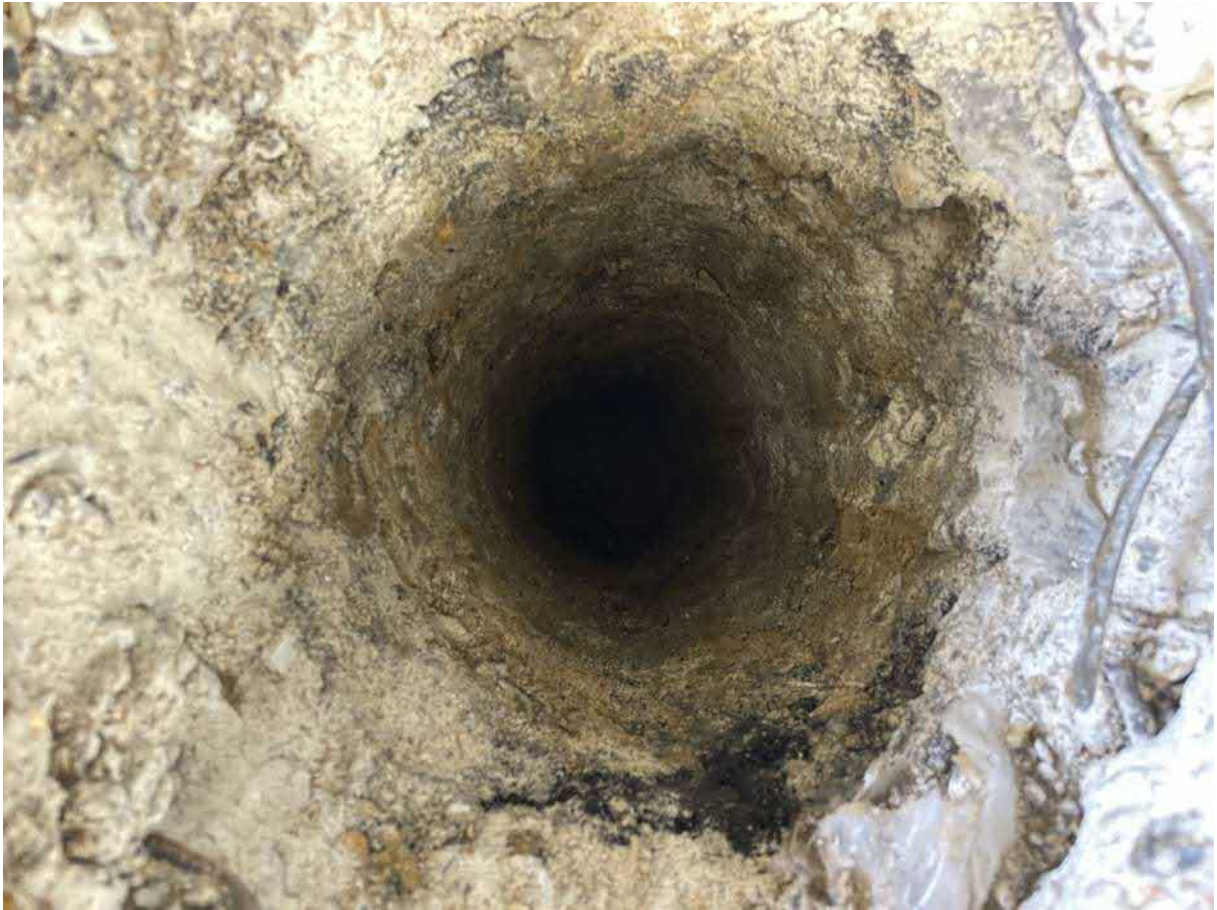
Photo 3—Example of a hand dug safety starter pit
