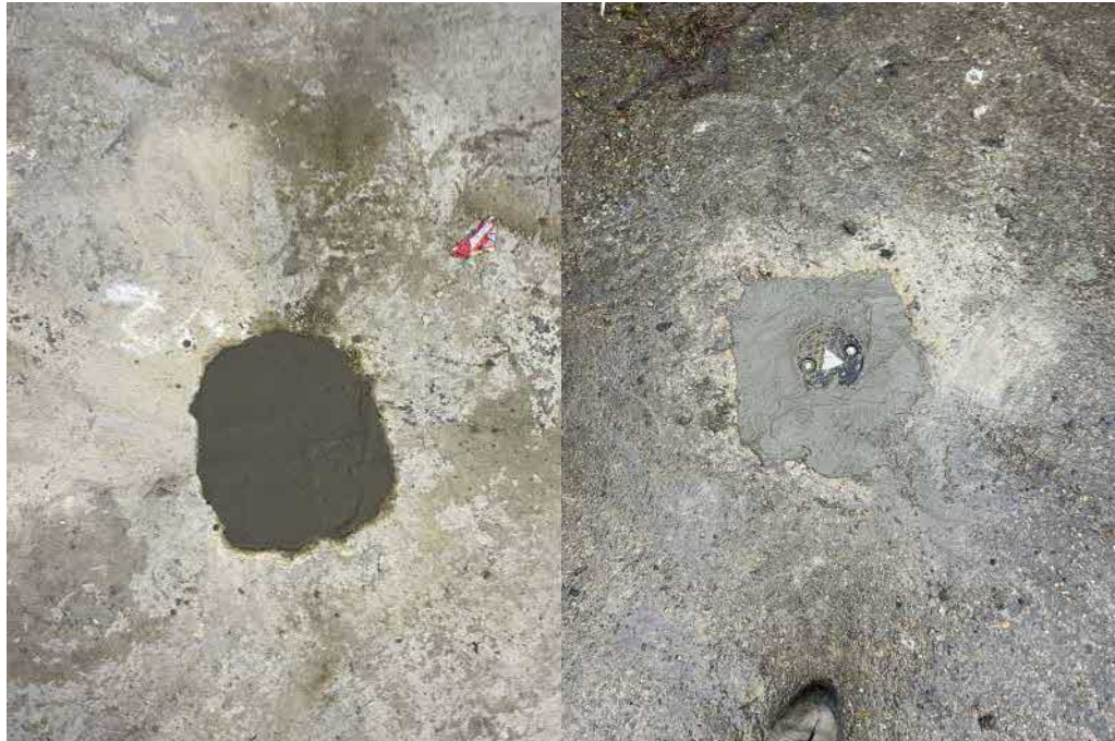
Photo 8—Examples of borehole reinstatement both with and without an installation
