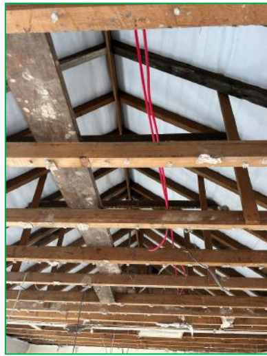
The internal roof structure of the northernmost structure.
