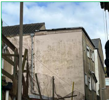
The flat-roofed extension.
