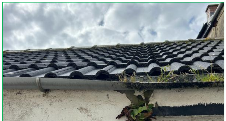
Showing tight-fitting tiles on the southernmost structure.
