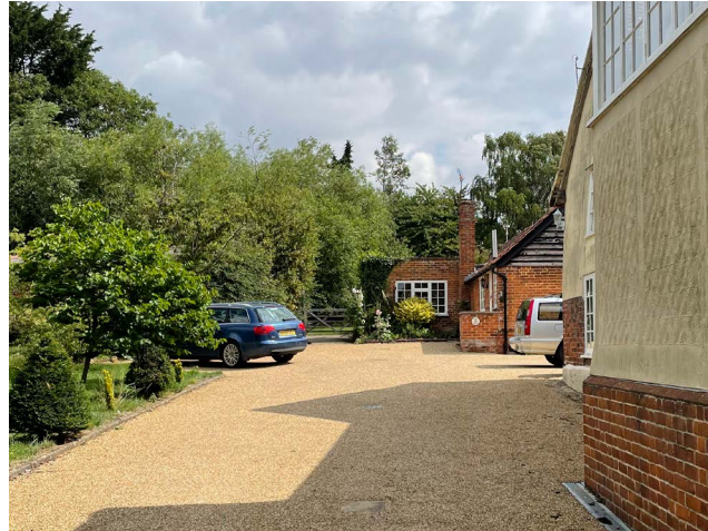
Wynne cottage as seen from driveway.
