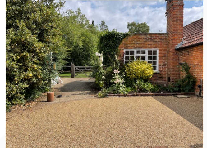
Previous addition to Wynne Cottage to be removed.
