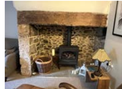
Fig 22: Fire place opened up
