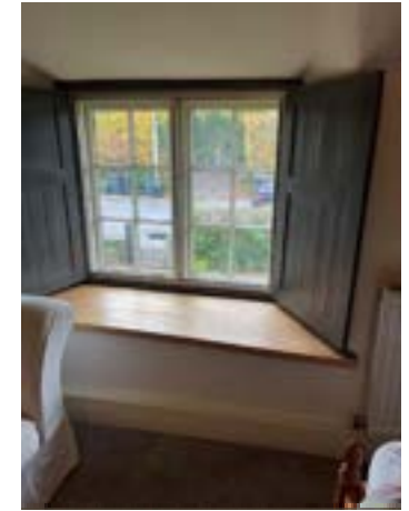
Fig 21: Replacement window board
