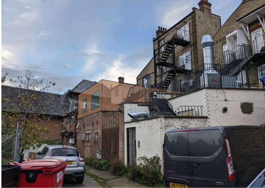
View of the rear of the property with rear extension indicated for scale.
