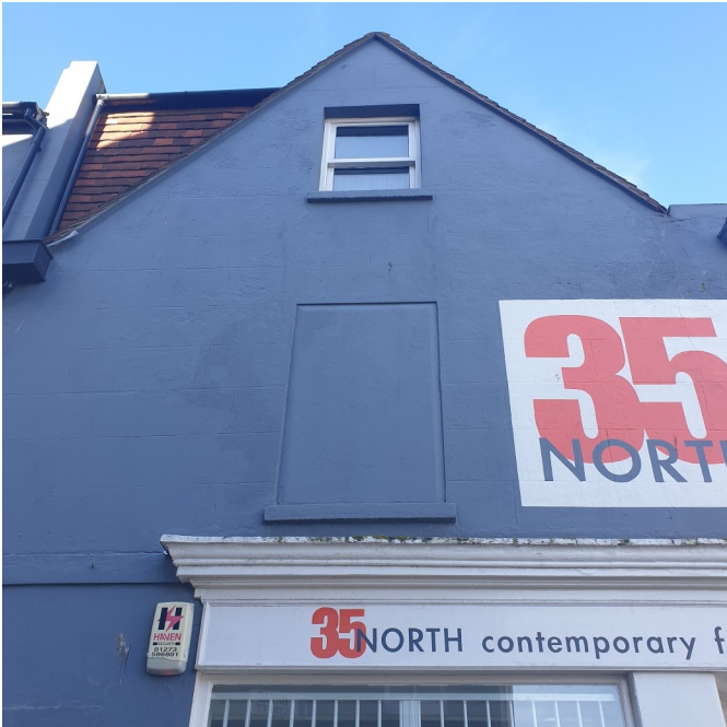
EAST ELEVATION DETAIL SHOWING BLOCKED WINDOW
