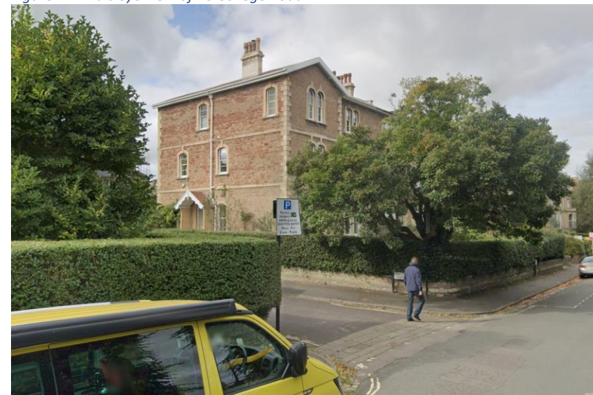
Figure 2 - view of 10 College Road from College Road
