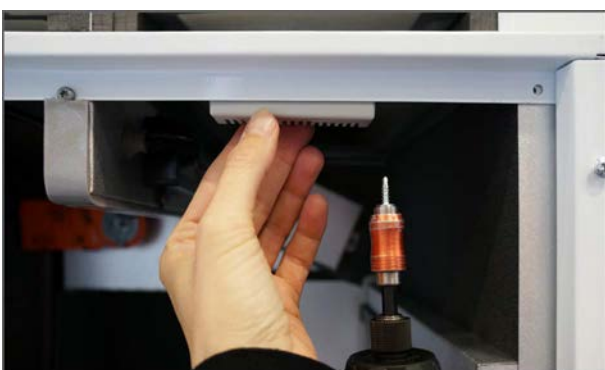
5. Mount the CO 2 sensor in the top cover, using self-threading screws (included in the CO 2 sensor kit).
