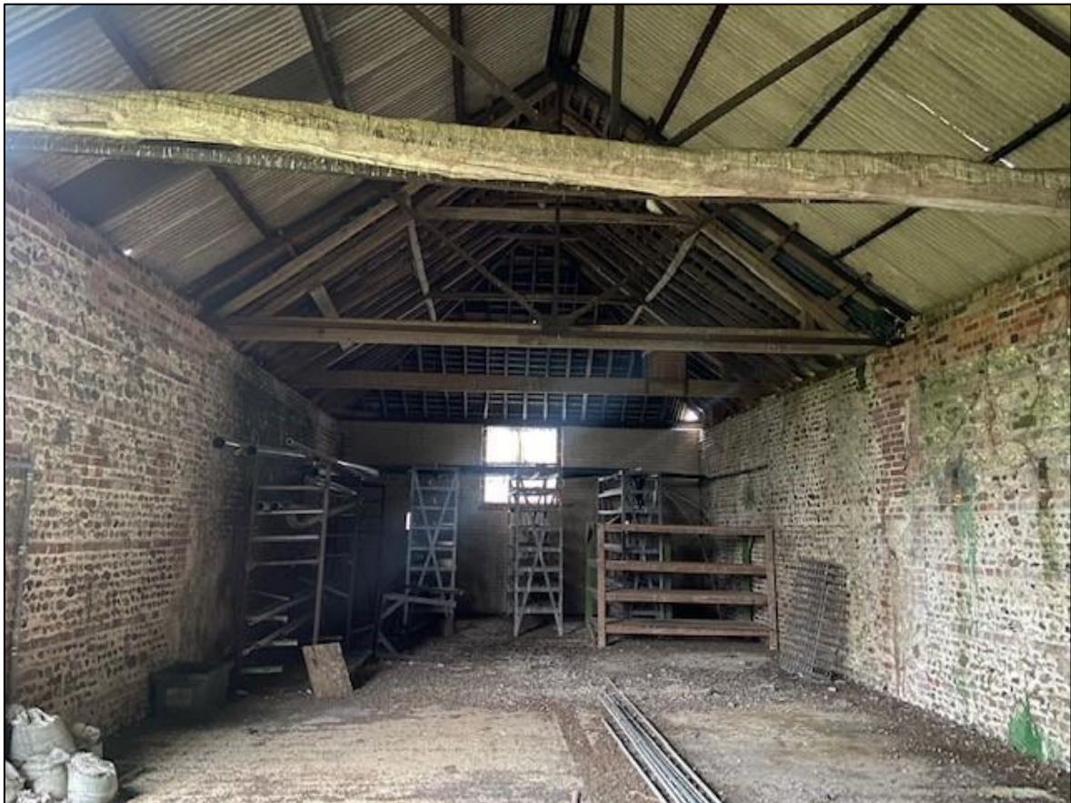
Internal structure (central barn, facing east)
