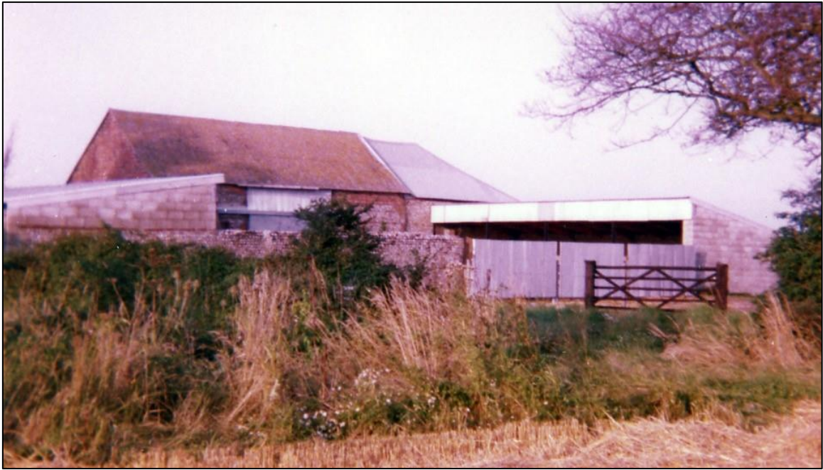
Historic photograph (photographed from the south-west)
