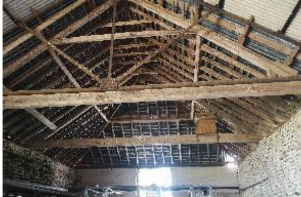
Figure 11. Internal view of the barn (taken June, 2022).
