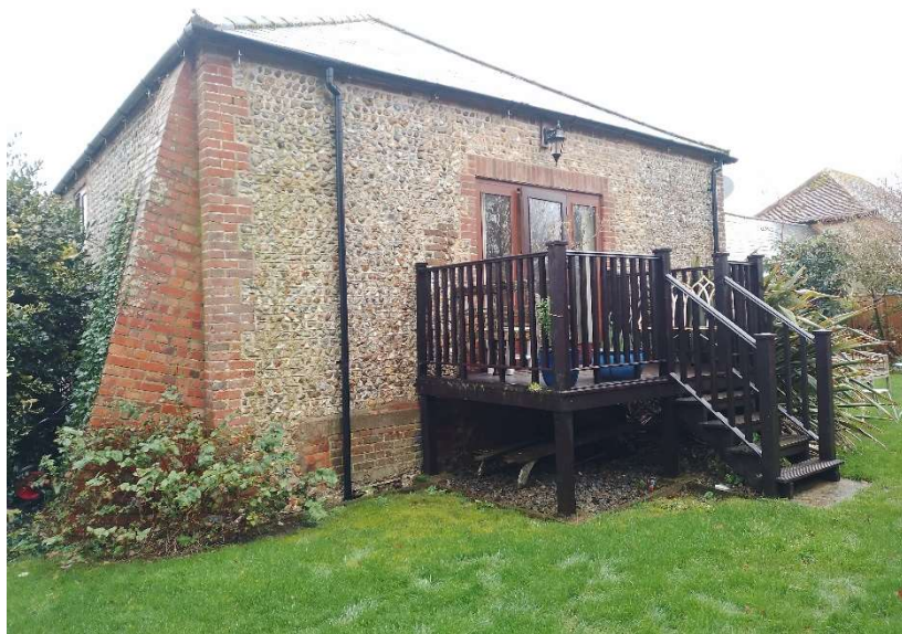
Existing raised external decking at Stumps Barn
